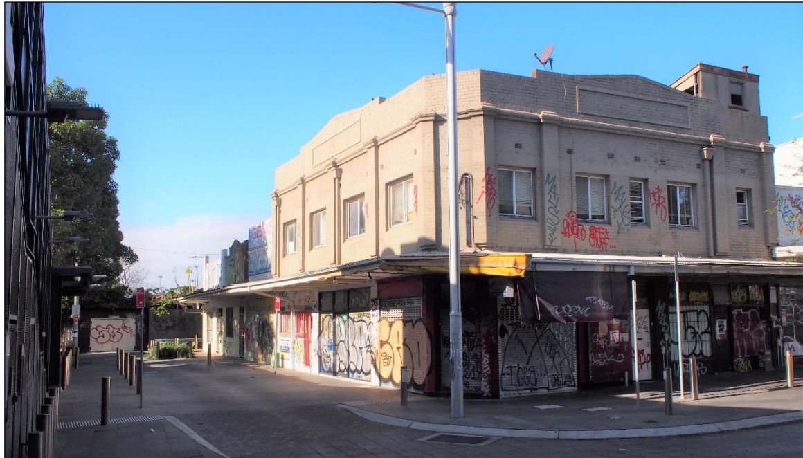
Figure 3: The site (to the right) opposite the Marrickville Railway Station.
