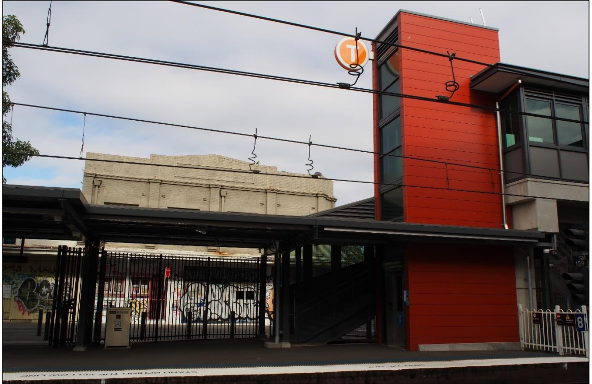
Figure 11: The northern part of the site viewed from Marrickville Railway Station..
