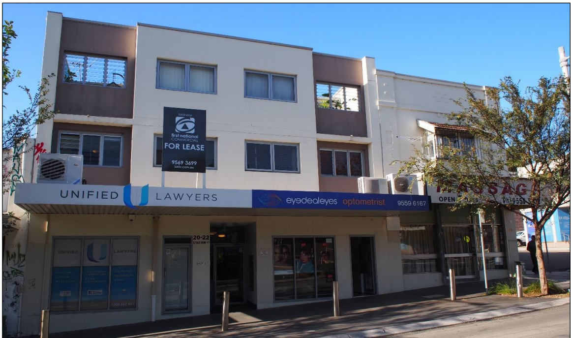
Figure 5: Three storey building at Nos. 20-22 Station Street adjacent the site to the south.
