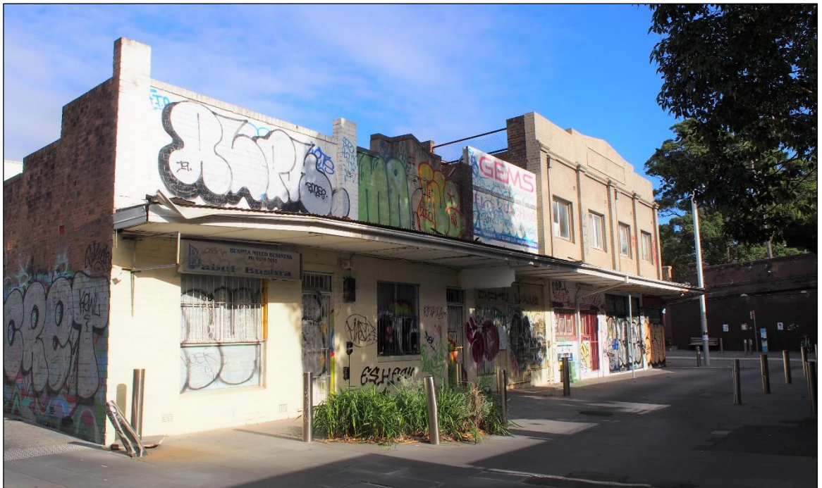
Figure 10: The north-eastern corner of the site viewed from Marrickville Railway Station.
